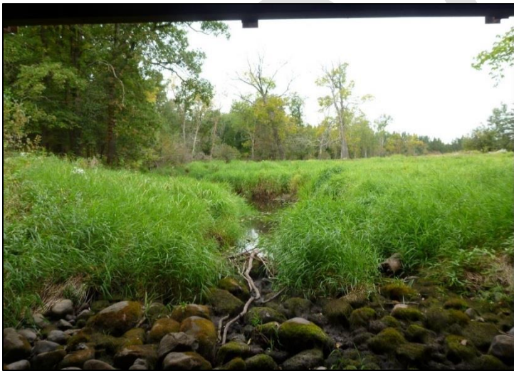
Figure BLANK (Left): Looking upstream from CR 196 bridge. The cobbles added during bridge construction were set at too high of an elevation. Water flows subsurface through cobbles, and the improper crest elevation of the cobbles is creating a flat water surface upstream. (Right): The coarse cobble substrate and lack of water underneath the CR 196 bridge.
