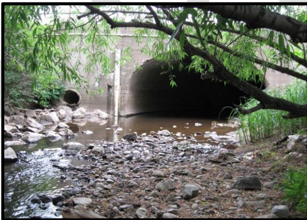
Figure 22c. Miller Creek outflows from an underground culvert that daylights at 26 th Avenue West in Duluth, MN. This culvert is not perched, but is representative of the habitat loss present in the urbanized setting.
