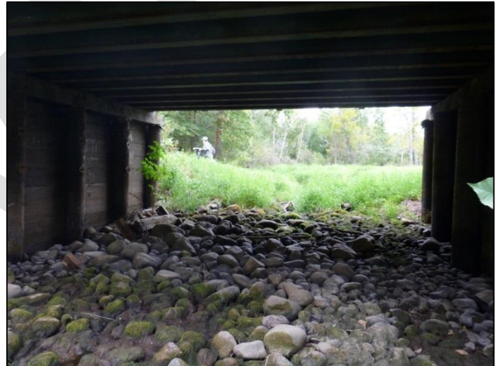
Figure BLANK (Left): Looking upstream from CR 196 bridge. The cobbles added during bridge construction were set at too high of an elevation. Water flows subsurface through cobbles, and the improper crest elevation of the cobbles is creating a flat water surface upstream. (Right): The coarse cobble substrate and lack of water underneath the CR 196 bridge.
