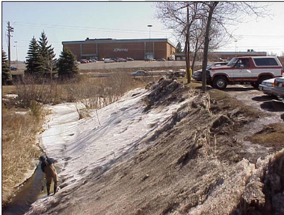
Figure 78: Large snowbank from a shopping center parking lot adjacent to Miller Creek. These snowbanks can contain significant amounts of road deicing salts and grit (sand/sediment). Photo Credit: Tom Estabrooks, MPCA- Duluth.
