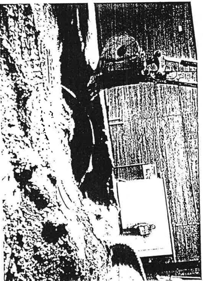
Photo 37. Owatonna Junior High--Purging and Uncovering Tank No. 8 and Tank No. 10
