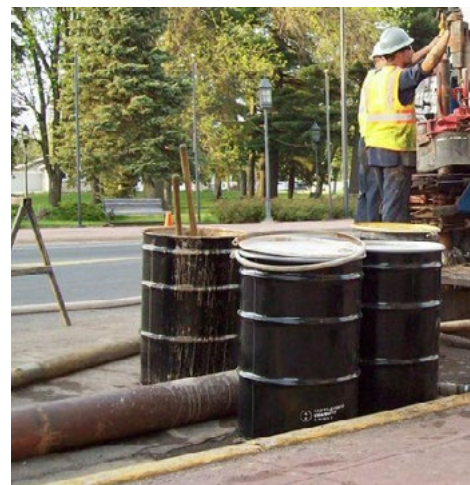
Rotosonic Drilling Waste, Biwabik Assessment, Biwabik, MN
