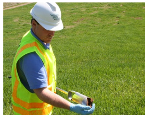
Soil boring to determine soil characteristics at Crow Wing Landfill
