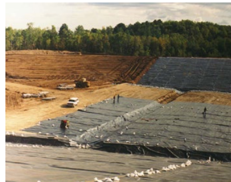
Crow Wing County Landfill liner installation observation
