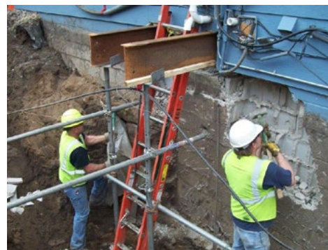
Observing State Contractors, Mitigation Project
