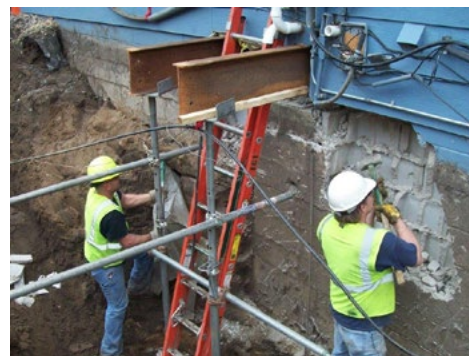
Observing State Contractors, Mitigation Project Hutto Residence, Anoka, MN
