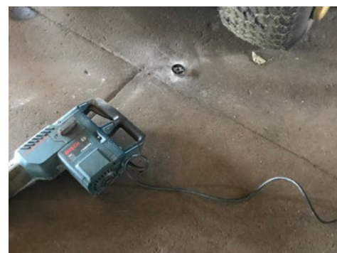
Vapor pin installation
