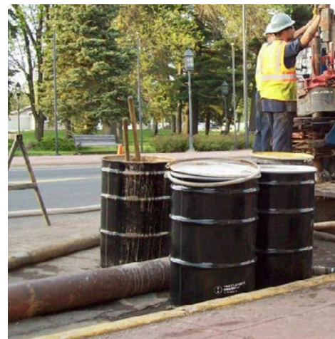
Rotosonic Drilling Waste, Biwabik Assessment, Biwabik, MN
