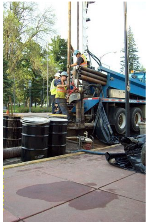
Rotasonic Drilling for City of Biwabik Assessment
