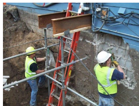
Observing State Contractors, Mitigation Project
