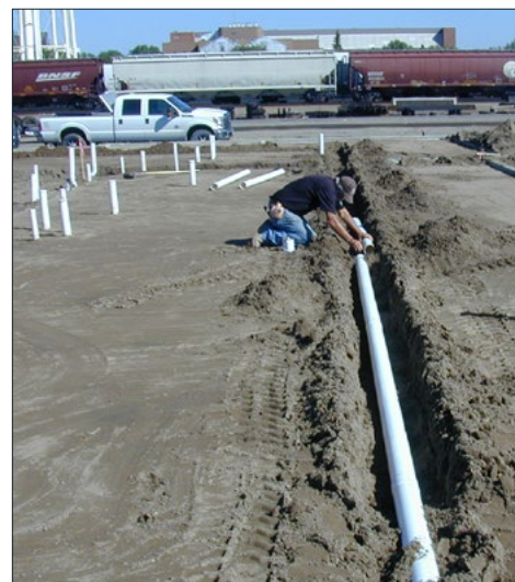
Completion of Approved Response Action Capital Solutions Site, Grand Forks, ND
