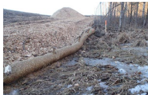
Construction Stormwater Inspection—MN TH 371, Nisswa, MN
