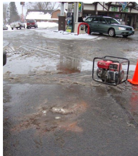
Installation of Passive Soil Gas Monitoring Canisters Biwabik Site Assessment, Biwabik, MN
