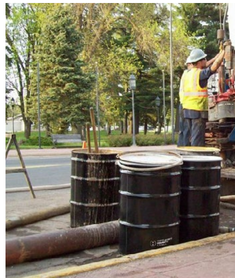
Rotosonic Drilling Waste, Biwabik Assessment, Biwabik, MN
