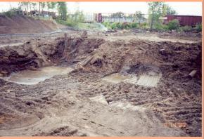
the material. A total of 46,000 cubic yards were excavated from two operable units of the site. Approximately 18,500 cubic yards of PCP contaminated soil were treated on-site. All but 2,850 yards met the on-site treatment criteria and were allowed to remain on site saving the MPCA the expense of off-site disposal.
