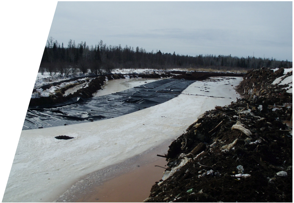
East Mesaba Closed Sanitary Landfill
