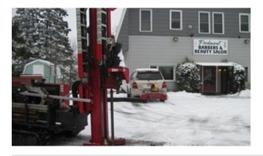
for the property to identify the extent and magnitude of soil and groundwater contamination at the site. The site had previously operated as a filling station, with tanks and dispensers located on the property. The tanks and dispensers had been removed at some time prior to current ownership, and the current owner was not aware of when the tanks and dispensers were removed. In addition, a small heating oil UST was removed from the site in December 1994.
