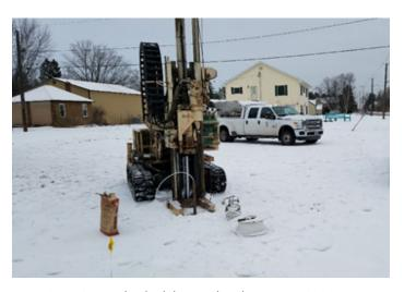
Vapor intrusion and sub-slab sampling has grown in importance over the past several years and MSA performs these activities on projects in both Minnesota and Wisconsin for petroleum and dry-cleaning contaminated properties.
