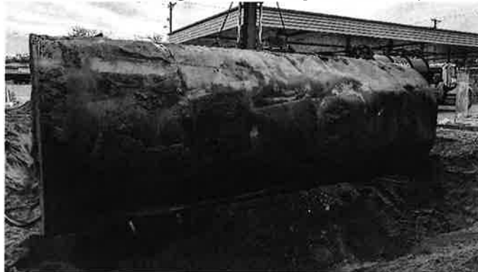
UST Removal oversight
