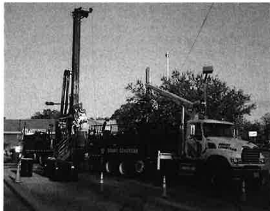
Rotasonic soil boring oversight
