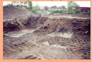
and screened. The contaminated soil was placed back in the excavation and a RCRA cap was installed over the material. A total of 46,000 cubic yards were excavated from two operable units of the site. Approximately 18,500 cubic yards of PCP contaminated soil were treated on-site. All but 2,850 yards met the on-site treatment criteria and were allowed to remain on site saving the MPCA the expense of off-site disposal.
