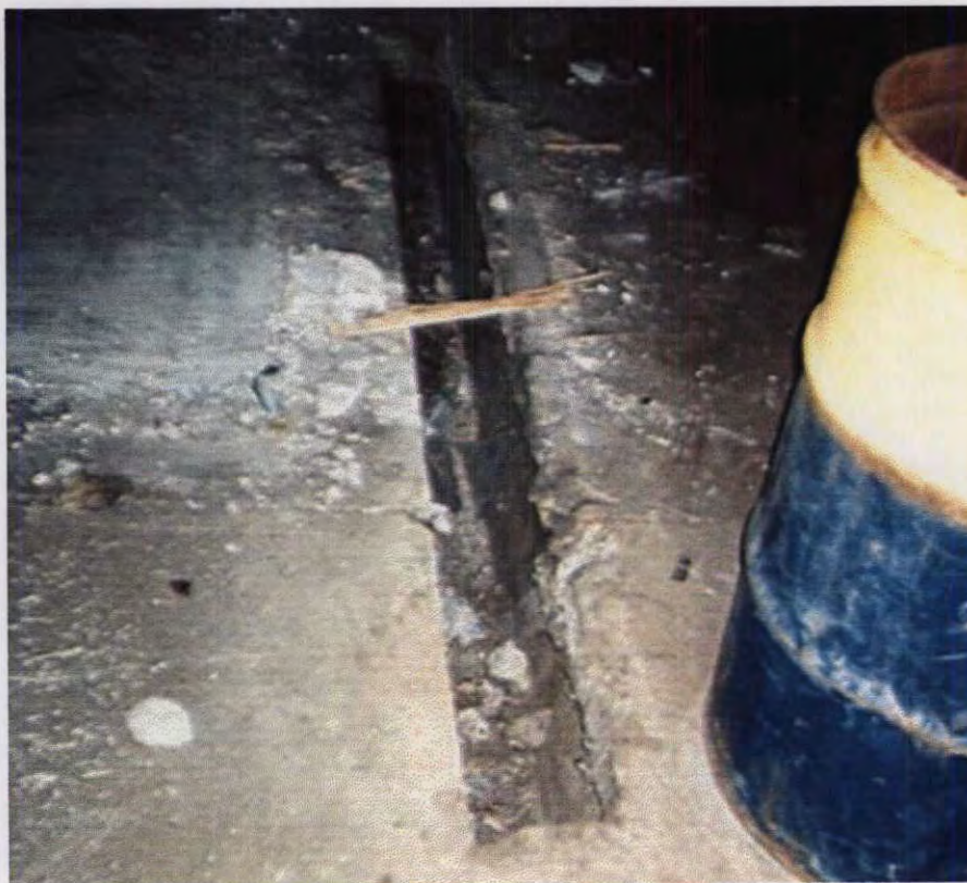
Photo 12 Floor Trench in the Former Alloy Hardfacing Building Area
