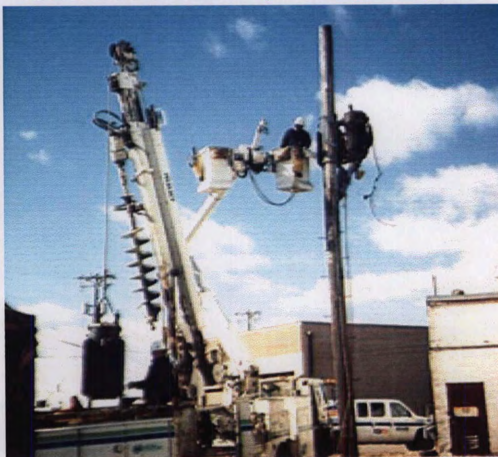
Photo 13 NSP Removing the Site Pole-Mounted Transformers
