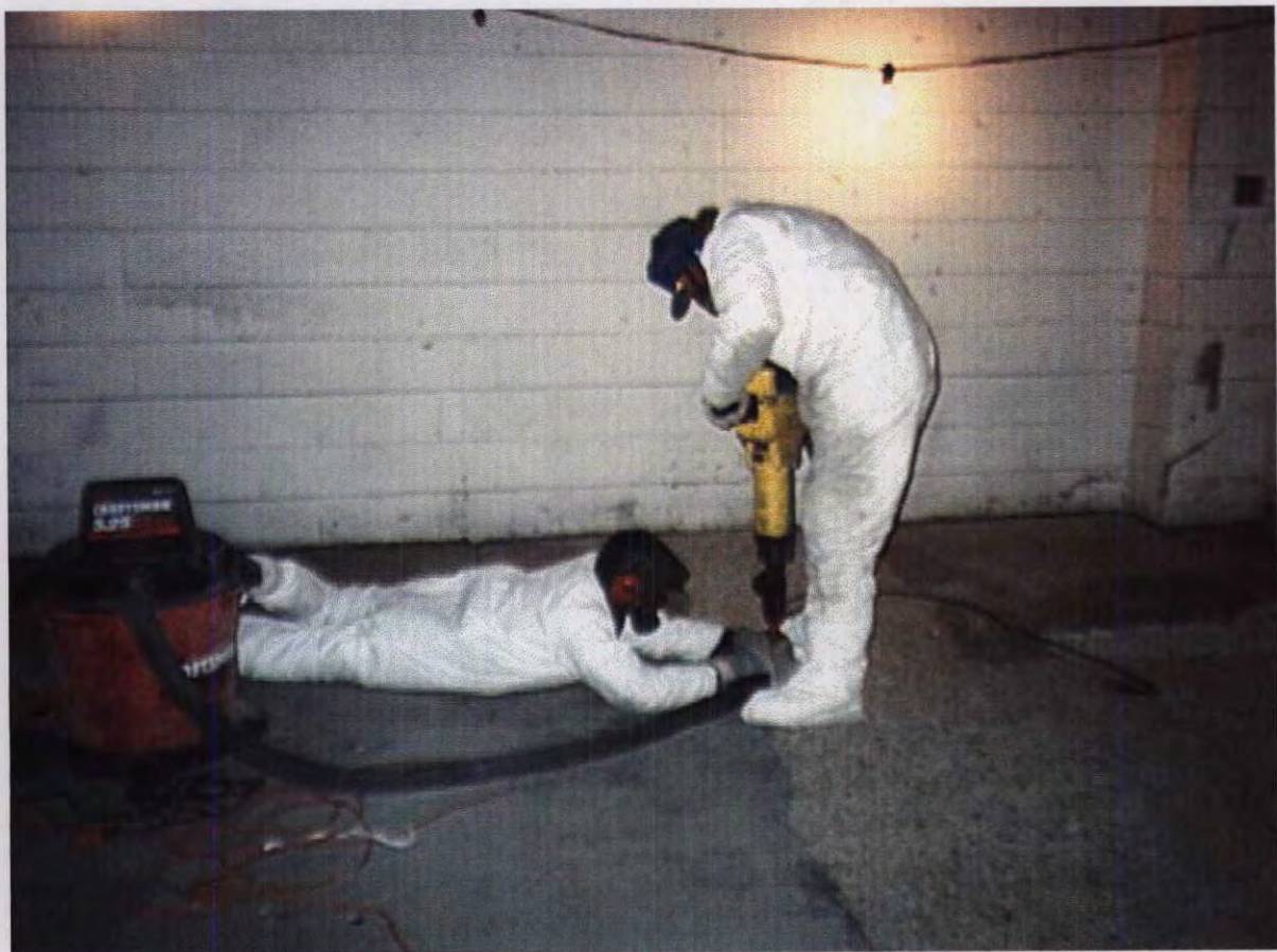
Photo 11 Scabbling PCB Impacted Concrete Inside the Former Alloy Hardfacing Building Area
