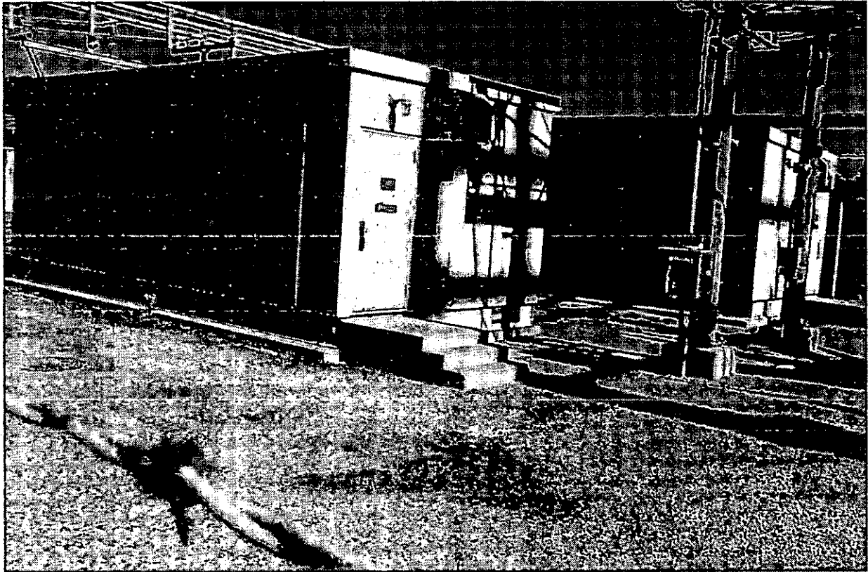
Photo 7 - View of two switch gear houses on the west side of the Site.
