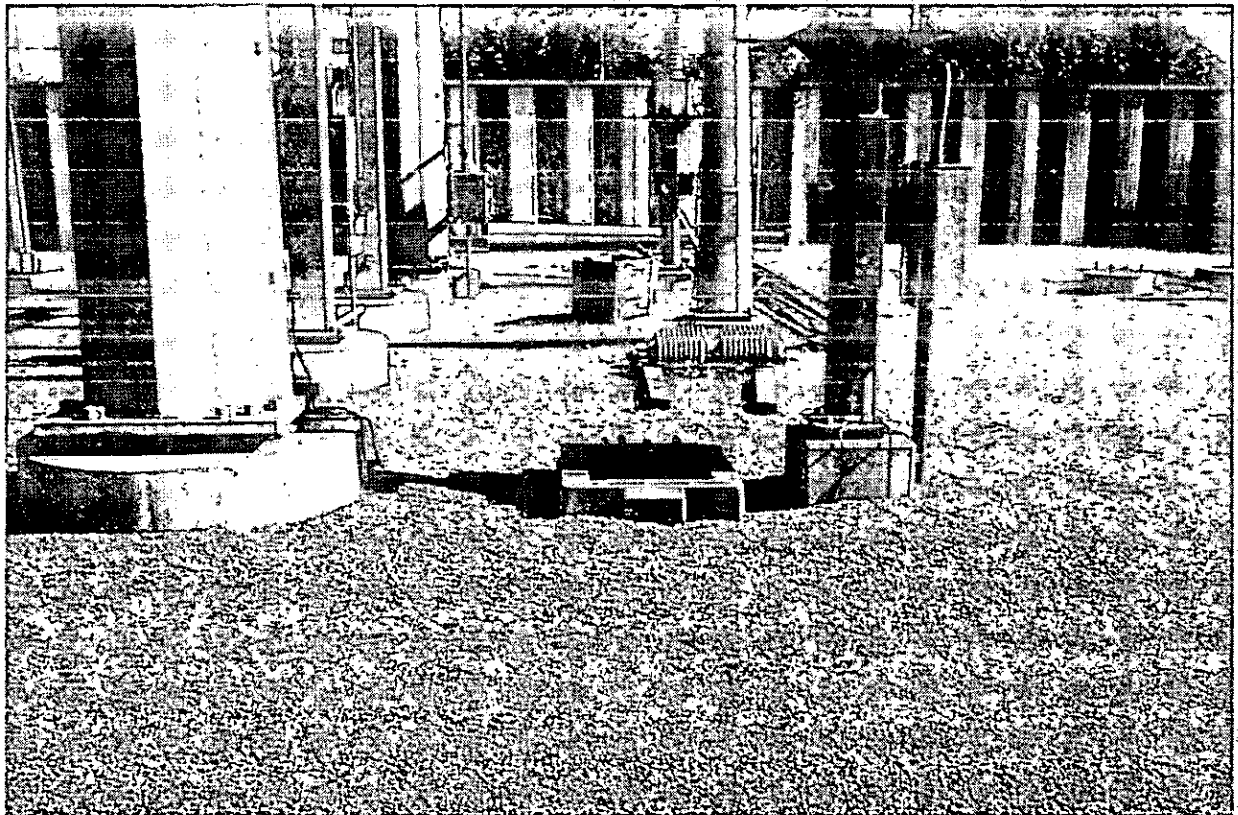
Photo 4 – View of small transformer base on the south side of the Site.
