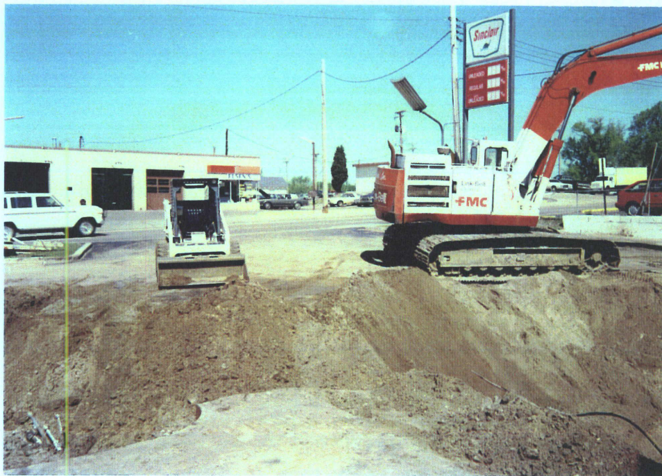
AREA BETWEEN THE PUMP ISLAND AND UST BASIN - NORTHWEST VIEW
