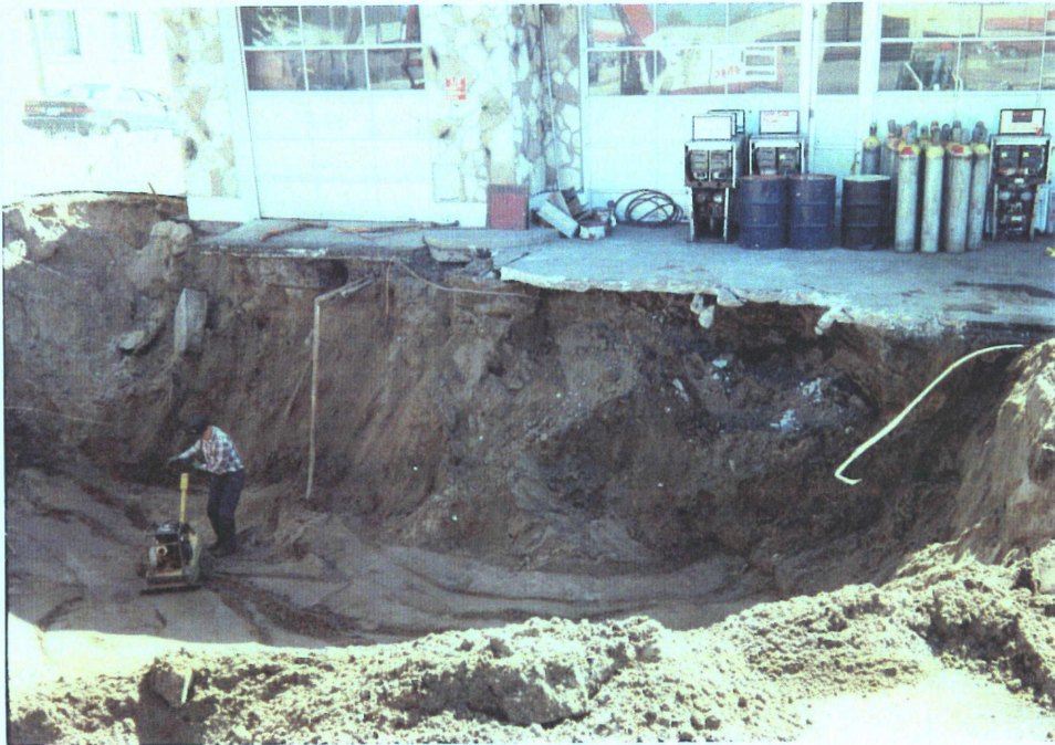
UST BASIN - EAST VIEW
