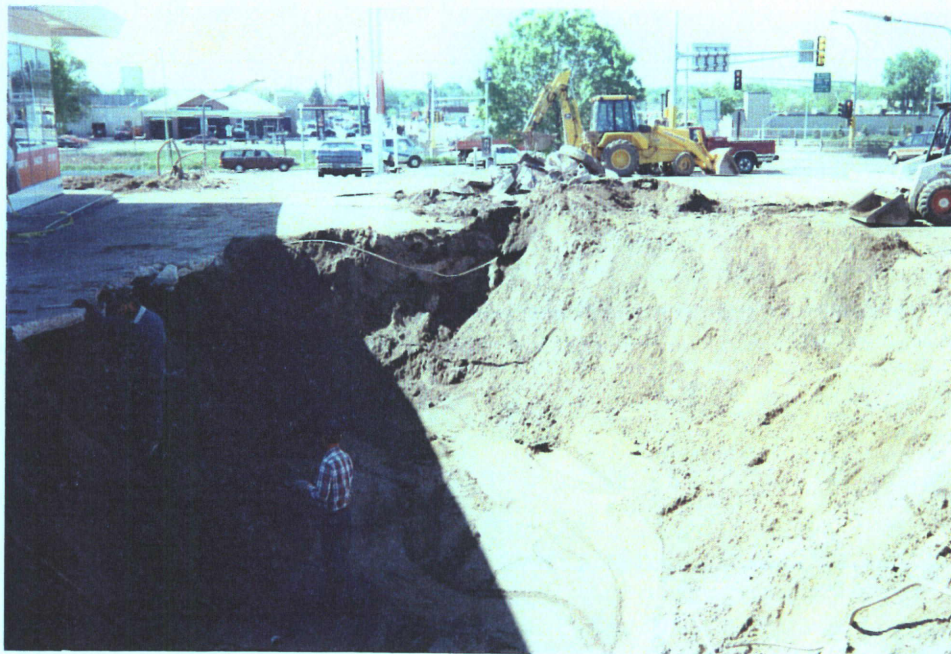
UST BASIN AND PUMP ISLAND AREA - SOUTH VIEW
