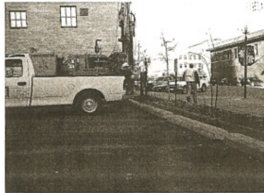
View looking north with drill rig set up on GB-2
