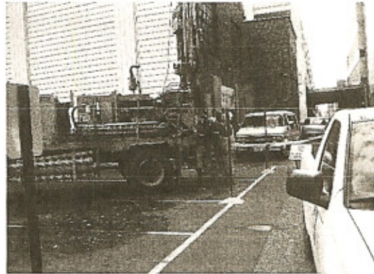
View looking west at drill rig set up on GB-1
