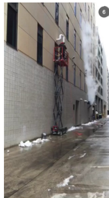
Scissor lift required to access stacks for pre-mitigation diagnostic testing.
