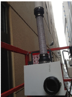
Pre-mitigation diagnostic testing pipe modifications with AMG Fury fan on top of scissor lift.
