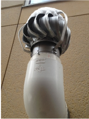
Close up existing rotary turbine ventilators connected to passive venting system.
