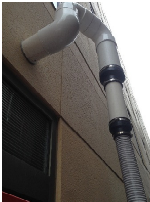
Pre-mitigation diagnostic testing pipe modifications.
