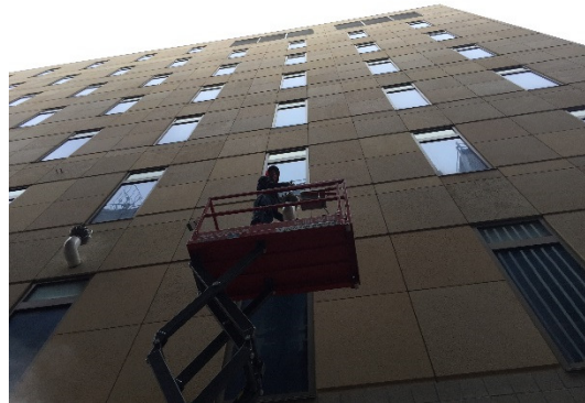
Scissor lift required to access stacks for pre-mitigation diagnostic testing.
