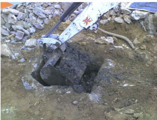
Source area pit excavation.
