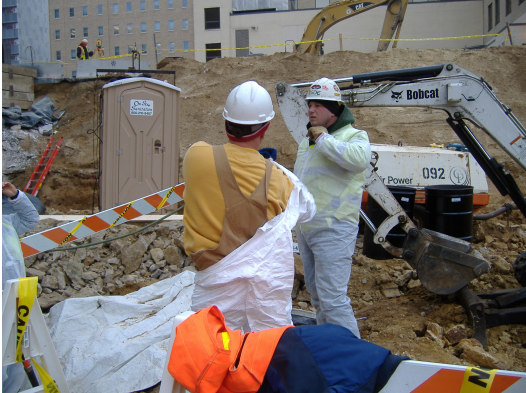
SDE and SWDI personnel donning PPE for HS-B7 hazardous waste removal.
