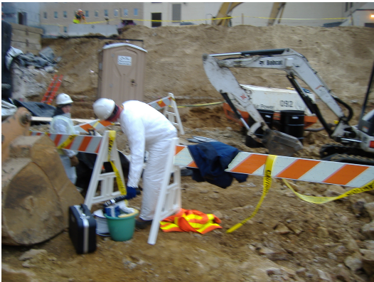
Landmark Environmental conducting air monitoring during HS-B7 soil removal.
