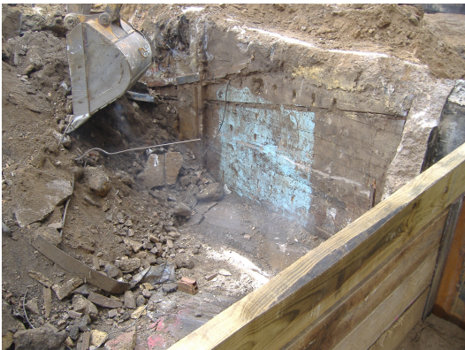
Photo looking southeast shows foundation wall bordering the south side of Parcel 223.
