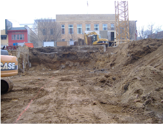
Photo looking east at remaining Parcel 223 foundation wall.
