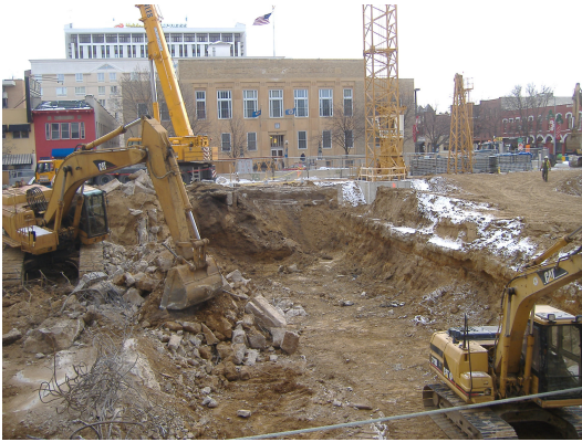
Photo looking east shows the Parcel 223 excavation area.
