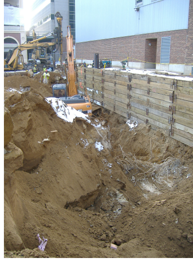
Photo looking south shows west side of parcel 219 excavation.
