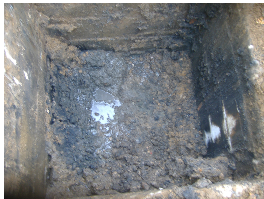
Photo looking inside of HS-B7 concrete structure.
