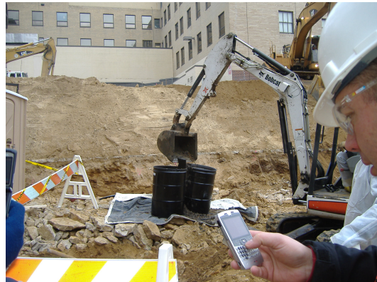
Filling barrels with impacted soils from source pit.
