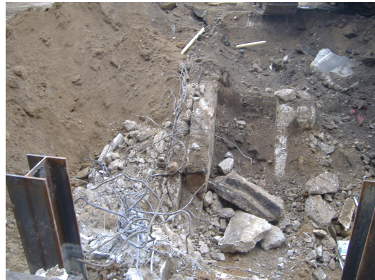
Photo looking east shows the foundation wall between Parcel's 223 (right) and 219 (left).
