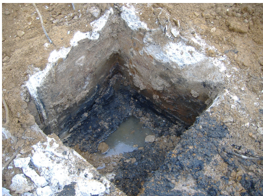
Depth of HS-B7 concrete structure as shown is 4 feet..
