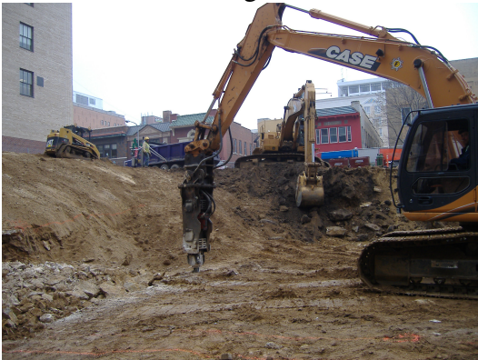
Photo looking east shows additional excavation activities at Parcel 219.
