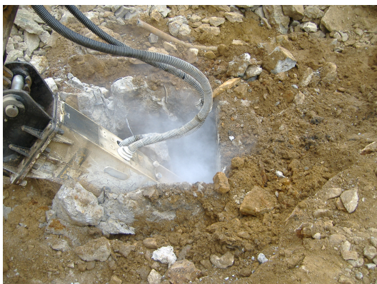
Hydro-hammer used for HS-B7 concrete structure and bedrock removal.
