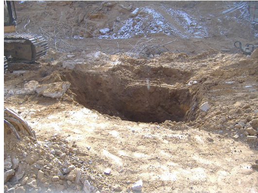
Photo looking north shows the initial B-7 area of concern excavation location.
