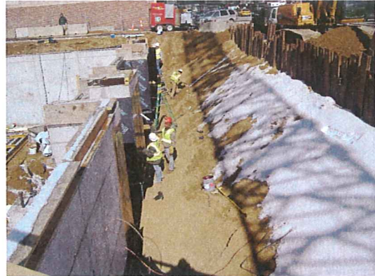
Feb. 26 and 27, 2008 - Extruding seams along the east side of the building
