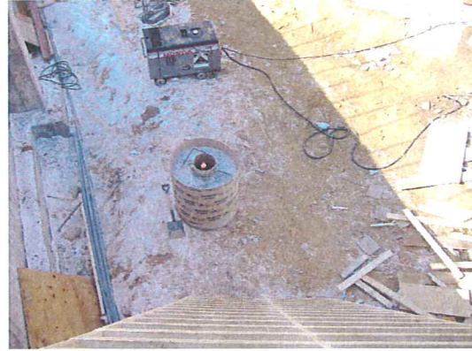
Feb. 5 thru 12, 2008 - Custom protective wellhead structure
