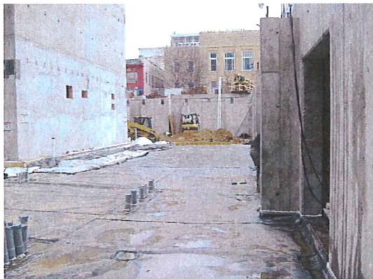
Mar. 25, 2008 – Additional vapor barrier installation activities
