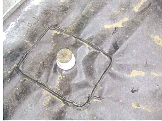
Mar. 25, 2008 – Completed vapor barrier pipe boot and extrusion welding
