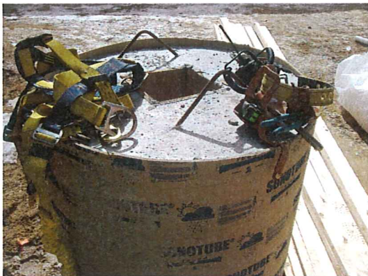
Feb. 26 and 27, 2008 - Custom protective structure
