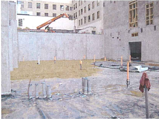
Mar. 25, 2008 – Additional vapor barrier installation activities
