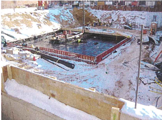
Mat slab vapor barrier installation.
