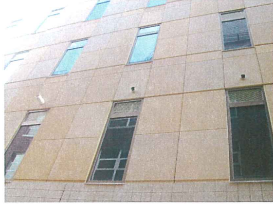
Passive venting (on left), DPE pump, and air stripper riser piping exiting the building
