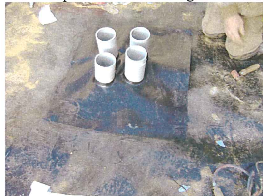
Mar. 19 and 20, 2008 - Another example of skilled hand work in sealing conduits
