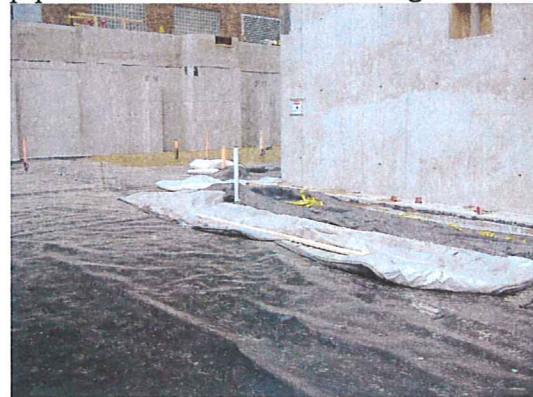
Mar. 25, 2008 – Additional vapor barrier installation activities
