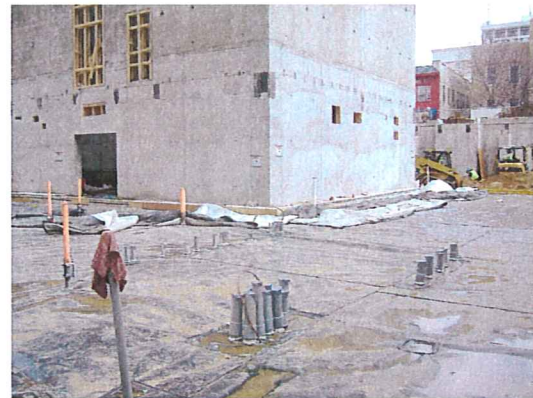
Mar. 25, 2008 – Additional vapor barrier installation activities
