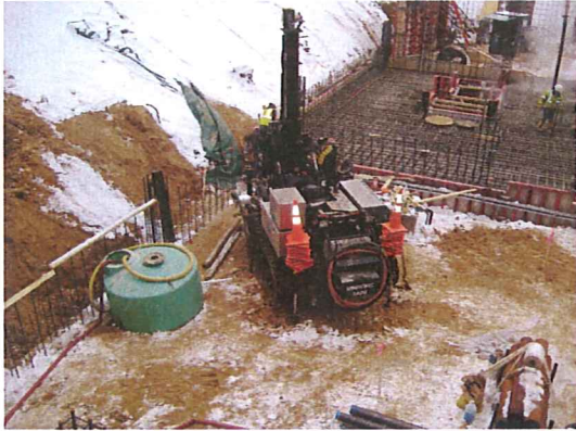
Feb. 5 thru 12, 2008 - Roto-sonic drill rig set up at DPE-2 location
