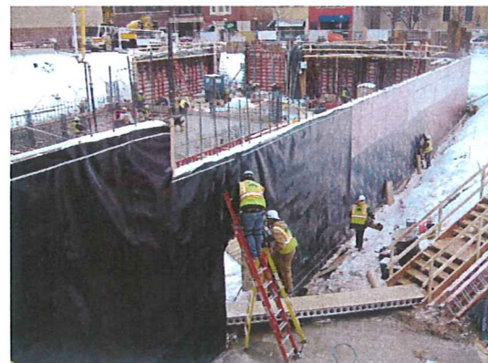
Vertical foundation wall vapor barrier installation
