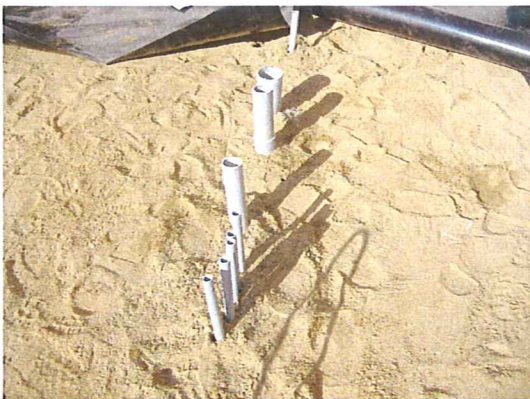
Mar. 19 and 20, 2008 - Bank of electrical conduit
