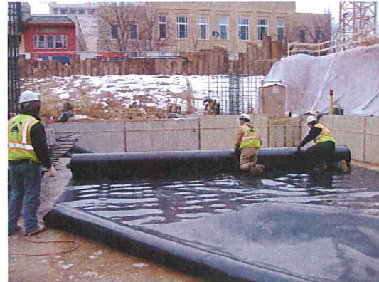
Mat slab vapor barrier installation.
