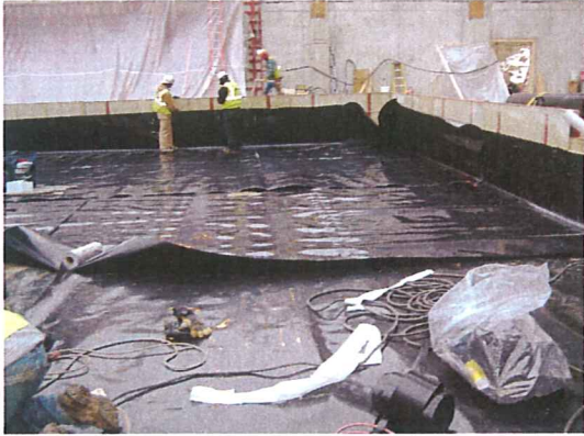
Mat slab vapor barrier installation.
