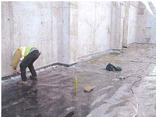
Mar. 25, 2008 – Additional vapor barrier installation activities
