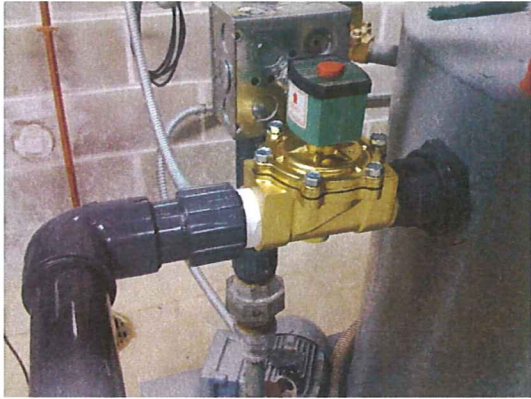
Solenoid valve between MS#1 and MS#2
