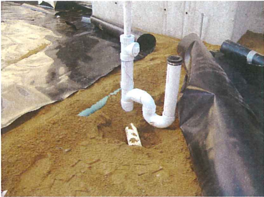
Mar. 19 and 20, 2008 - Future floor drain and venting system in foreground
