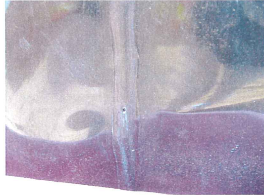
Feb. 26 and 27, 2008 - Typical extrusion seam
