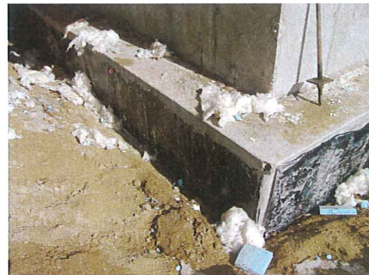
Feb. 26 and 27, 2008 - Existing vapor barrier under the super footing
