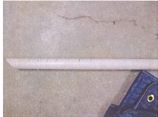
Slits cut into DPE system drop tube
