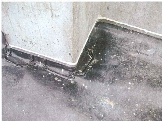
Mar. 25, 2008 – Completed vapor barrier connection to the vertical wall
