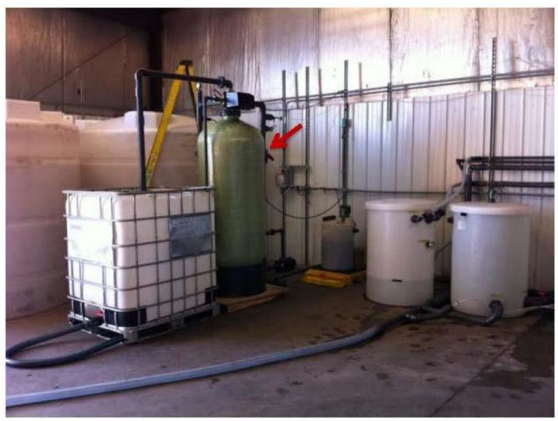
Figure 5 Greensand Filter Pilot Unit
