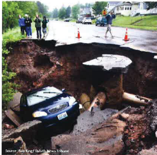
Flash Flooding creates sinkholes in roads, swallowing cars in Duluth, MN, 2012
