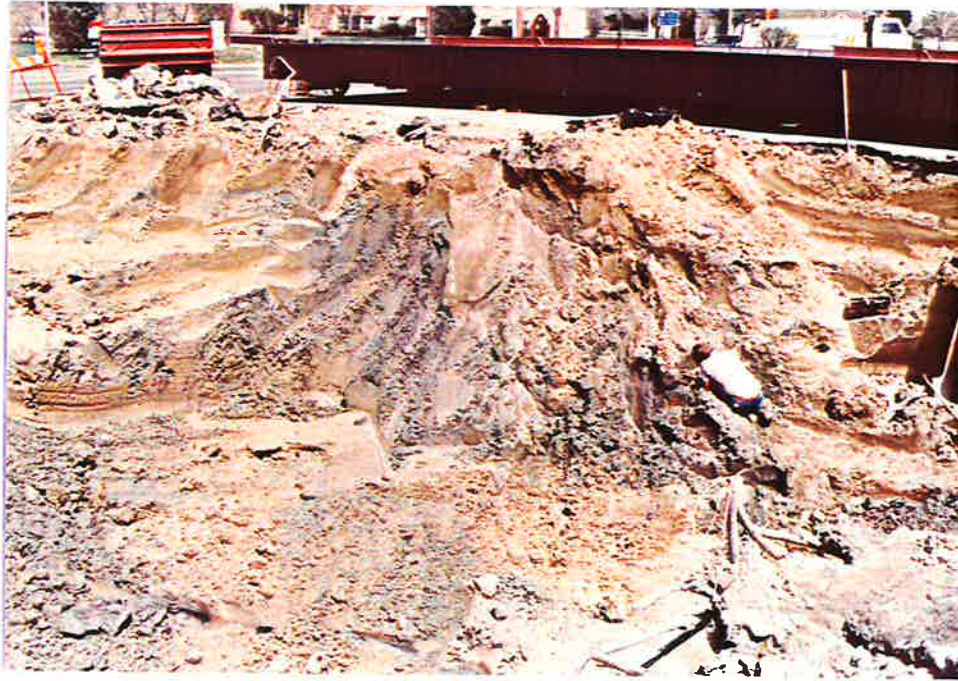
PHOTOGRAPH 5 EAST SIDEWALL OF EXCAVATION, REPAIRING WATER SERVICE
