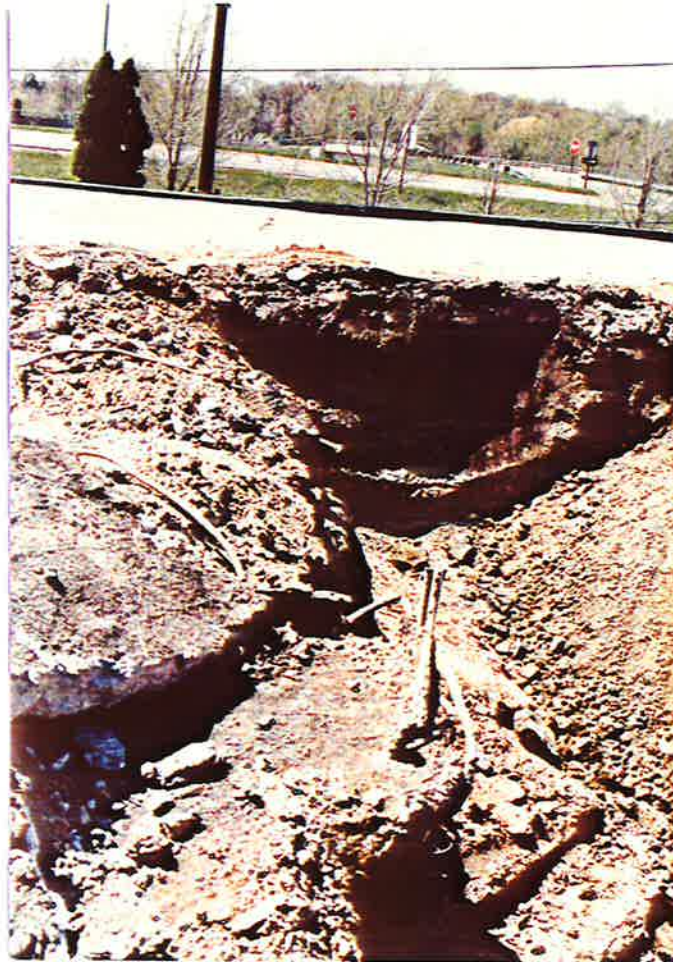
PHOTOGRAPH 7 WEST SIDE OF EXCAVATION, VIEW UNDER ROAD EASEMENT
