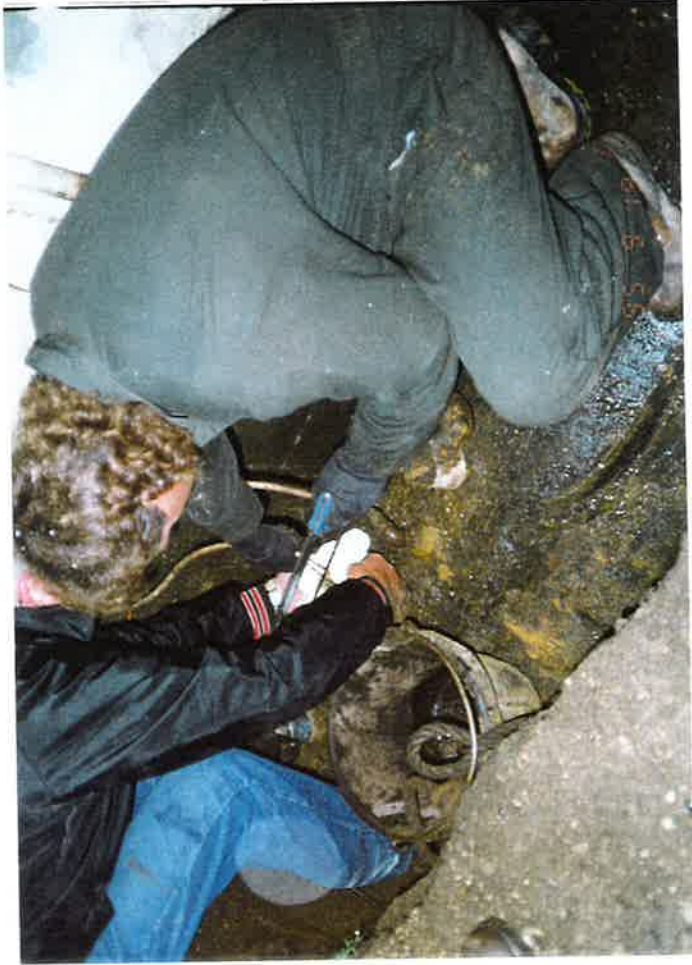
PHOTO NO. 2 Removal contractor cutting supply and return piping
