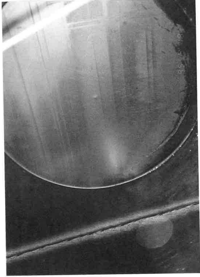
PHOTO NO. 8 View of cleaned inner tank lining
