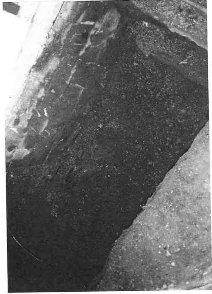
PHOTO NO. 7 Tank excavation base immediately following removal of UST
