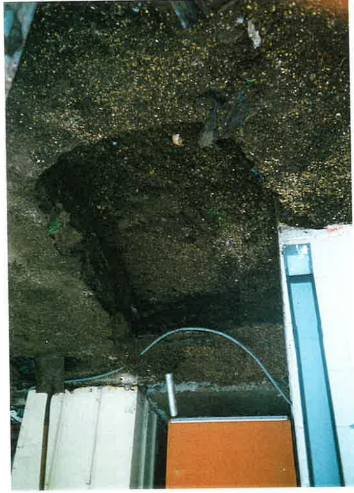
PHOTO NO. 10 Evacuation backfilled with existing soil
