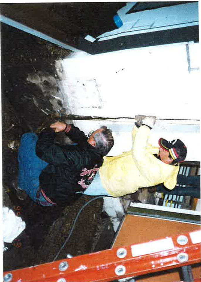
PHOTO NO. 3 Workers removing steel vent pipe
