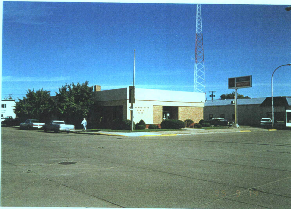
Photograph No. 14B: Northwestern State Bank LUST site.
