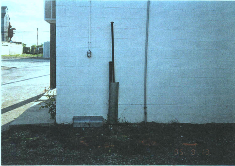
Photograph No. 1: Worksite prior to excavation activities.
