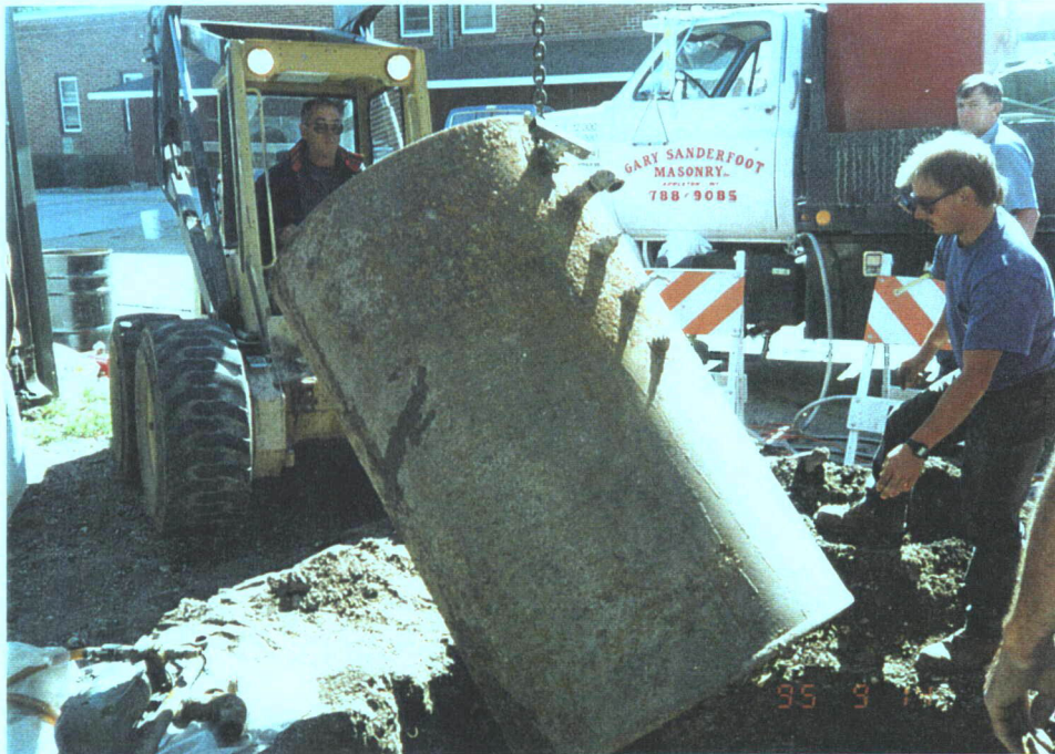
Photograph No. 6: Removal of UST from excavation.
