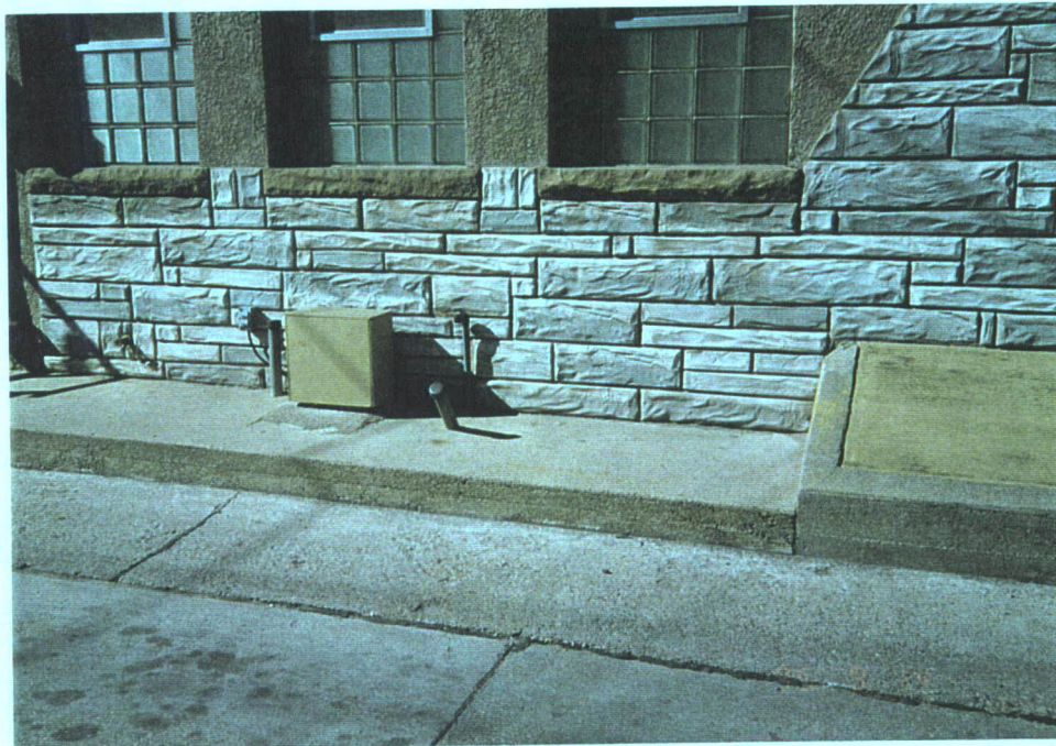
Photograph No. 14D: Gullander's Hardware possible UST vent and fill piping.
