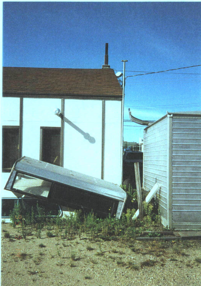
Photograph No. 14C: C&M Ford Body Shop UST vent location.
