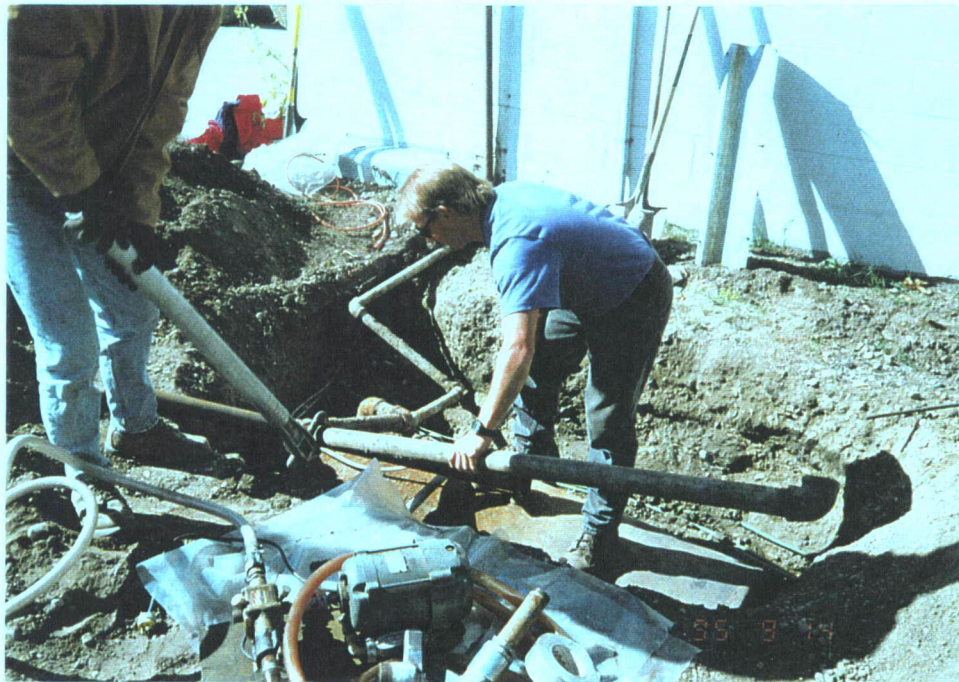
Photograph No. 4: Workers disconnecting fill and vent piping.
