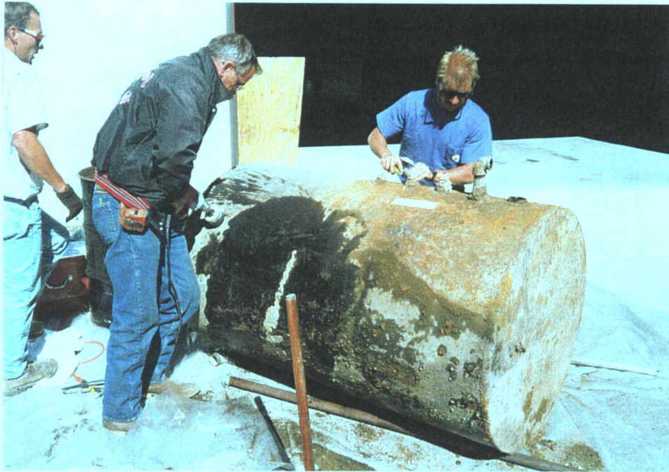
Photograph No. 11: Worker cutting open tank sidewall.
