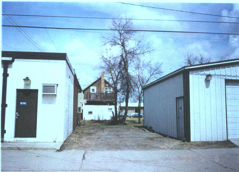
Photo #2 View of facility (looking north) showing location of overhead electric lines
