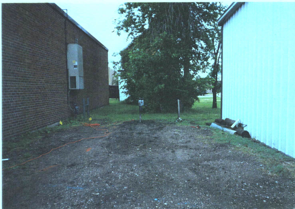
Photo #3 Set up at HA-SB-3. View of ESP set up.
