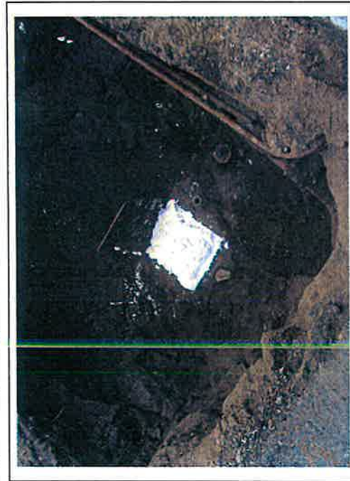
Facing: Into UST basin. View of: Foaming of in-place UST
