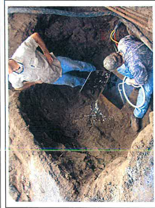
Facing: Into UST basin. View of: Foaming of in-place UST
