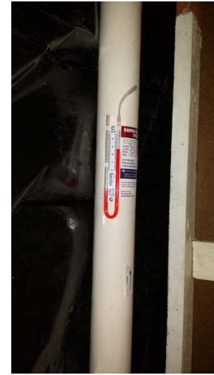
Photo 18: View of the system label and U-Tube manometer following final system set-up.
