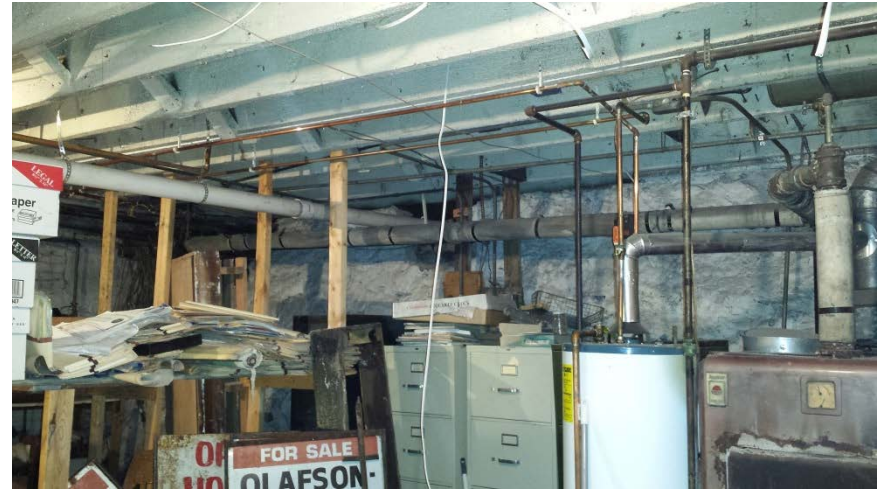
Photo 6: Attempting to depict the openings into the crawlspace that required sealing along the stone wall separating the basement from the crawlspace.
