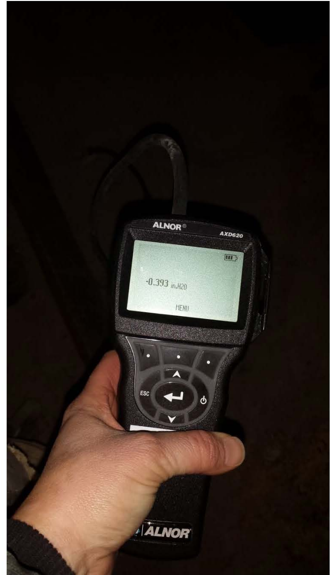
Photo 22: View of final mitigation system test point readings: TP-07 reading.
