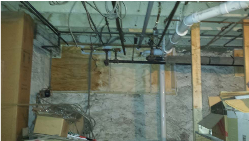
Photo 7: View of one of the openings into the crawlspace following sealing.
