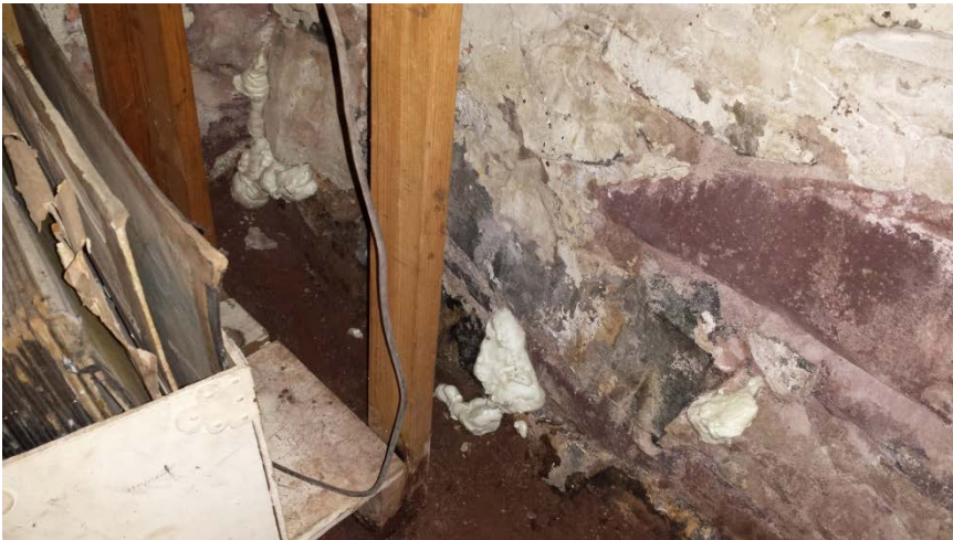
Photo 3: View of the gaps in the crawlspace wall following sealing.
