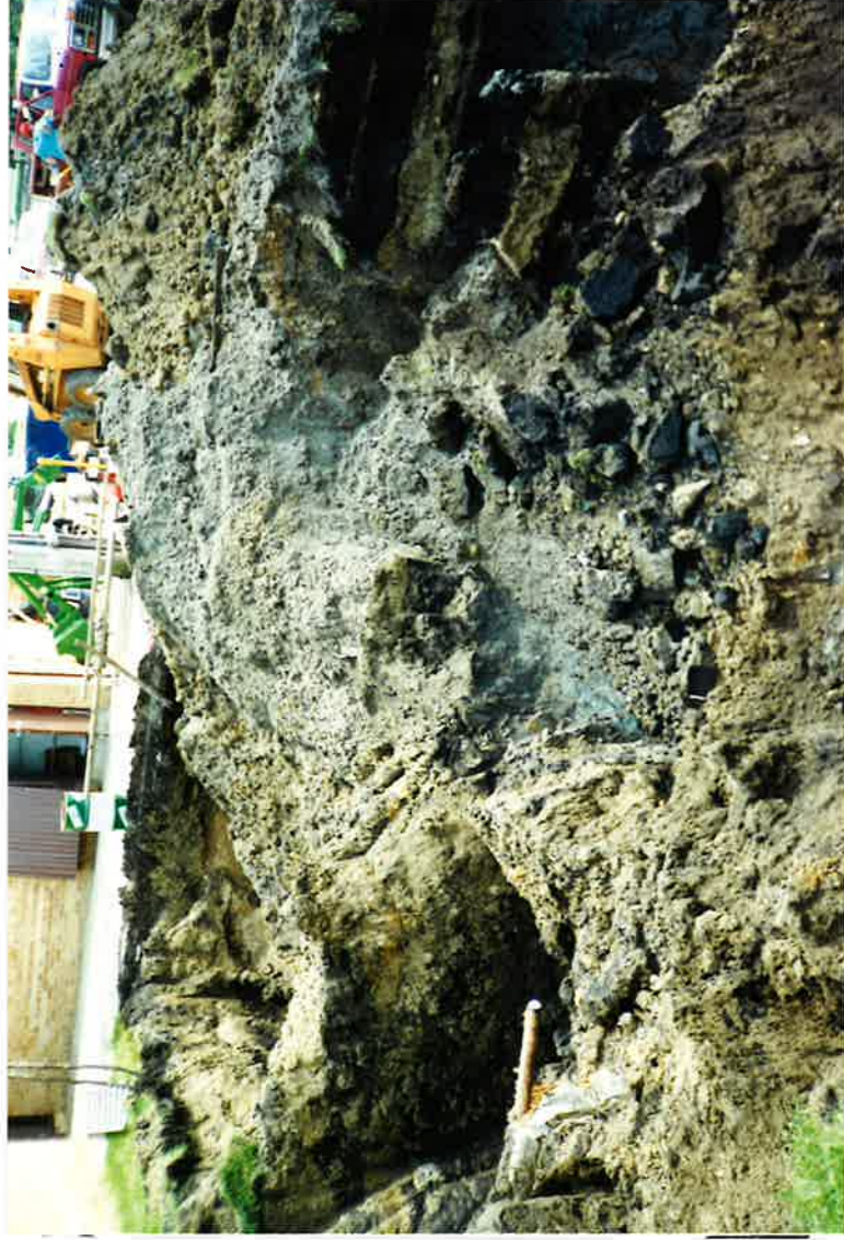
Martin County West High School Petroleum contaminated soil returned to excavation
