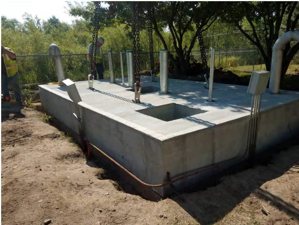
New vault cover installed.
