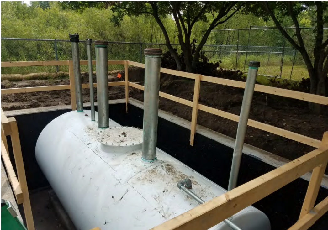
New tank and vent/access pipes installed.
