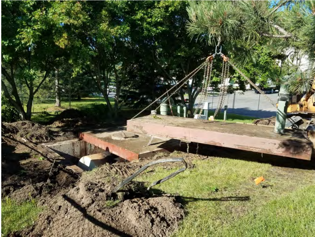
Removal of existing vault cover.
