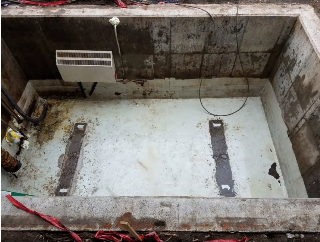
Tank removed, vault cleaned.
