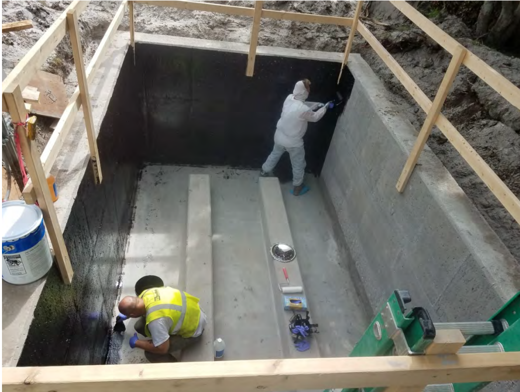
Concrete patched, grout poured on floor, CIM 100 sealant being placed.
