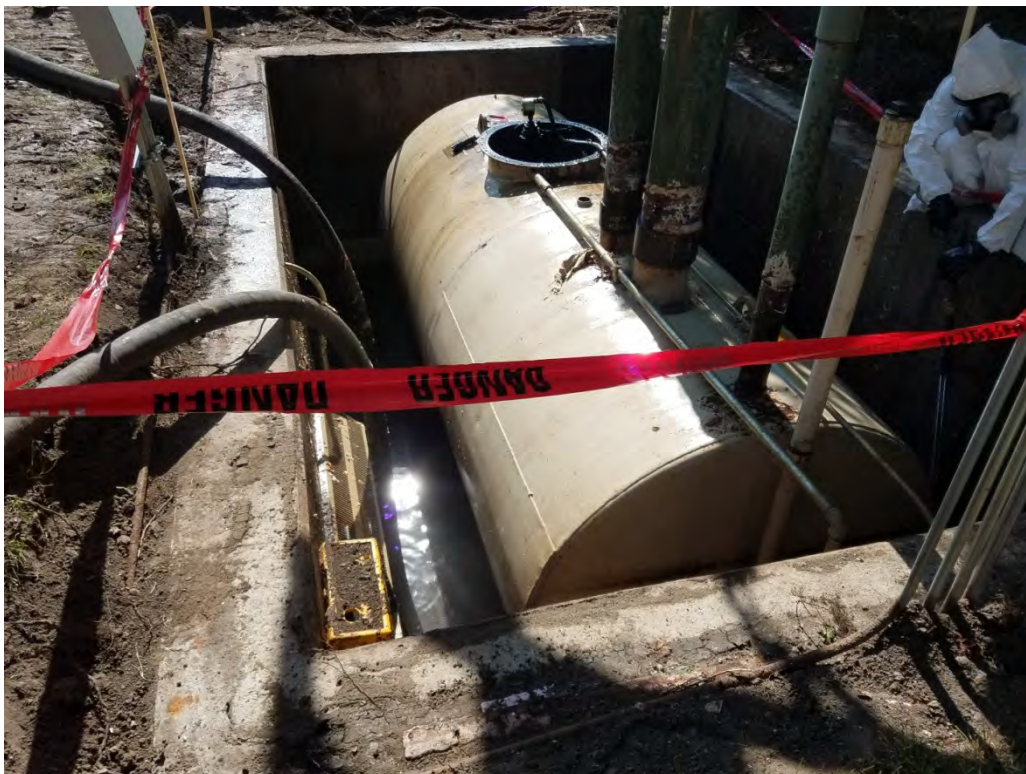
Old tank, vault cover removed, tank cleaned.
