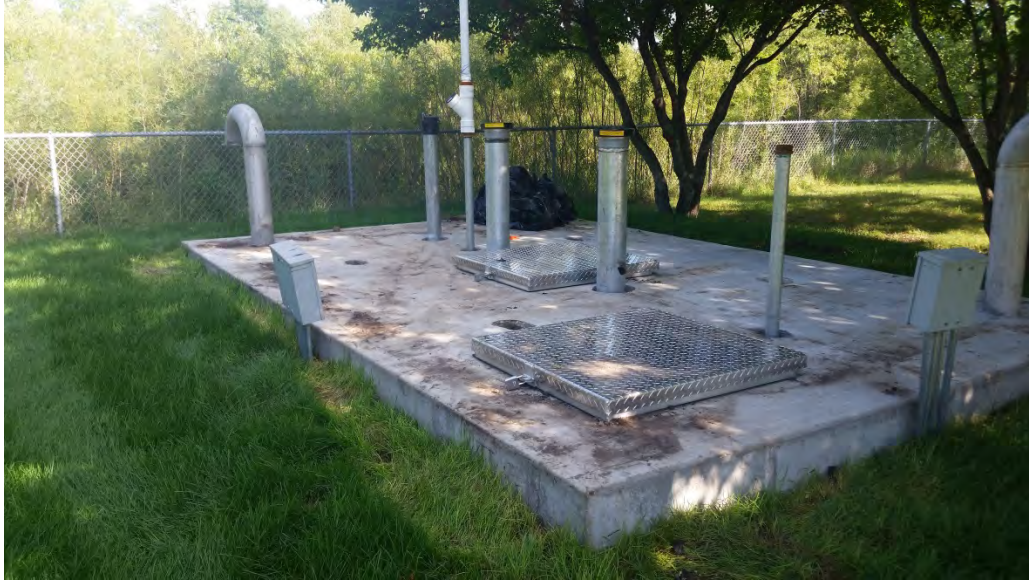
Vault cover in place, new sod placed.
