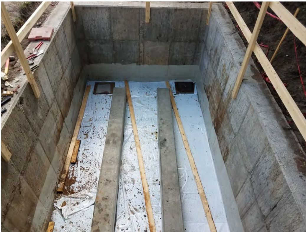
New footings poured.
