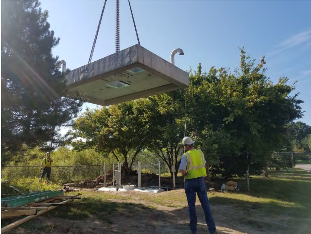
New vault cover delivered.
