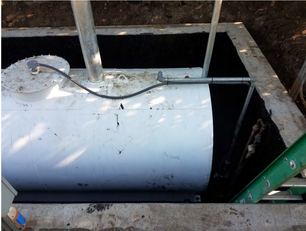
New high level float and wiring installed.
